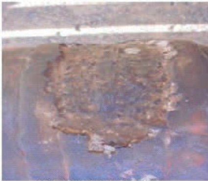
Spalling at Fusion Line
