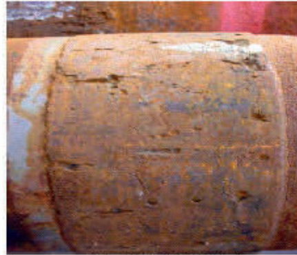
Spalling from Porosity
